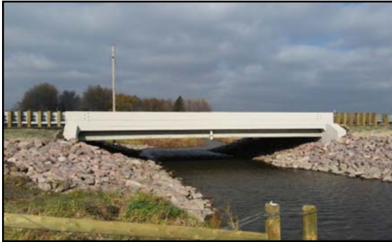
Minnehaha County Replacement Structure, Pre-stressed Inverted-T Girder with Composite CIP Deck. Submitted by Civil Design Inc.
