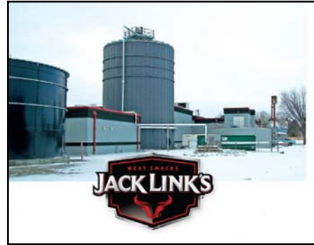
Link Snacks, Inc. (LSI) Wastewater Pretreatment Facility. Submitted by Banner Associates, Inc
