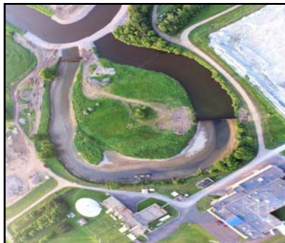
Elm River Intake Protection and Channel Improvements Water Treatment Plant. Submitted by Clark Engineering
