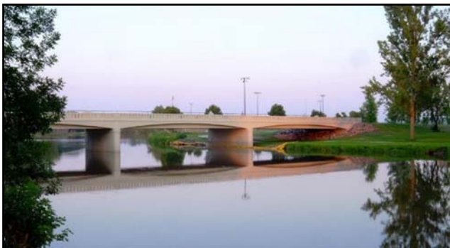
Garfield Avenue Bridge Replacement in Dell Rapids, SD. Submitted by SEH
