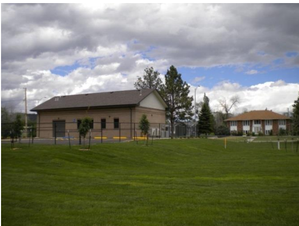
NORTH RAPID BOOSTER PUMP STATION PROJECT SUBMITTED BY BARTLETT & WEST
